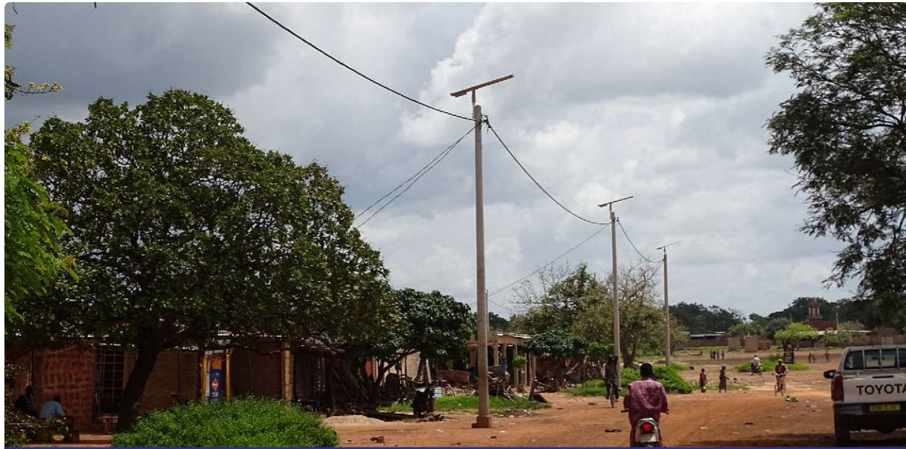
Rural electrification in the village of Kouakoualé, powered by FRES. UNCDF / Touré Monia Roxane
