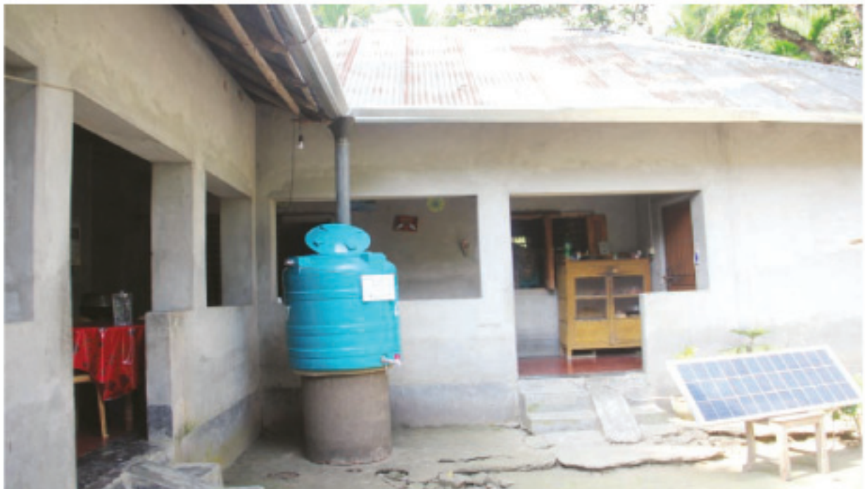
Rainwater harvester with model climate resilient community : photo ©Sajjadul/LoCAL-UNCDF
