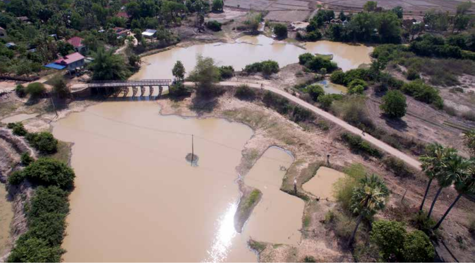
LoCAL-supported elevated road in Rokakiri District, Battambang, Cambodia; photo: Cédric Jancloes © UNCDF/LoCAL
