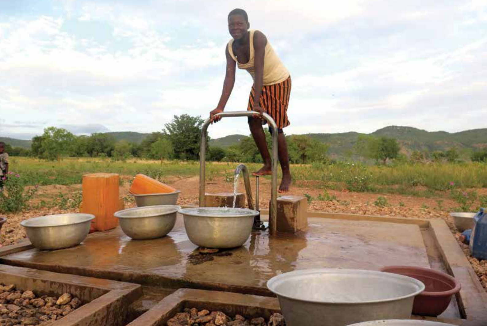
Foot pump, Boukoumbe, Benin; photo: Nasser Alqatami © UNCDF/ LoCAL
