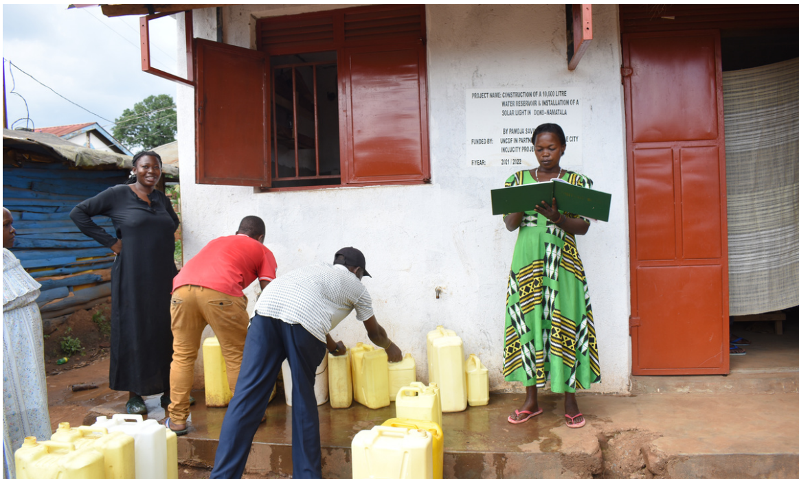
UNCDF-installed new water reservoir, Mbale City, Uganda Source: UNCDF.
